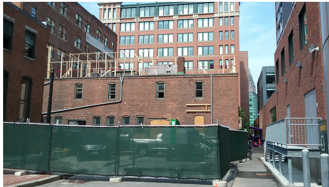
VIEW 2 - FROM MBTA VENT STACK
