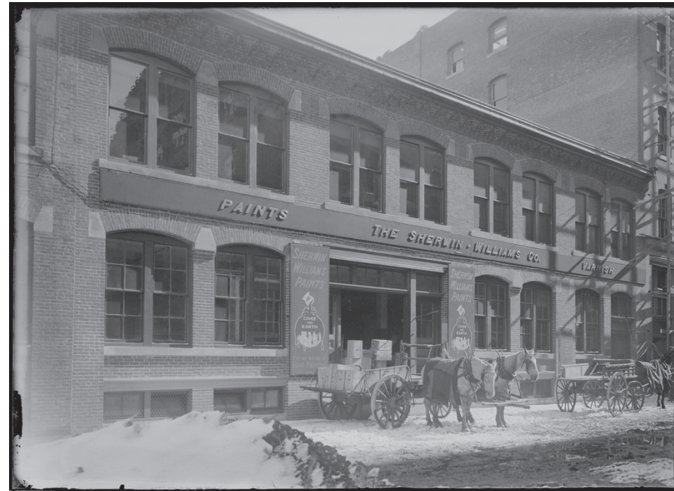
SIGNAGE BAND & SIGNAGE NEXT TO ENTRY DOOR
