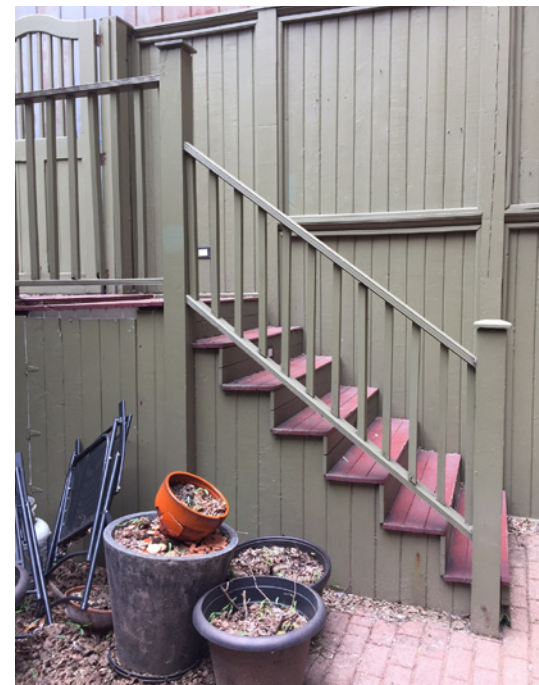
Existing stair to be replaced
