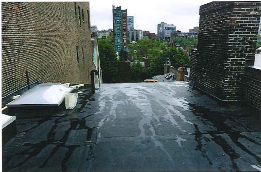
South Facing View
