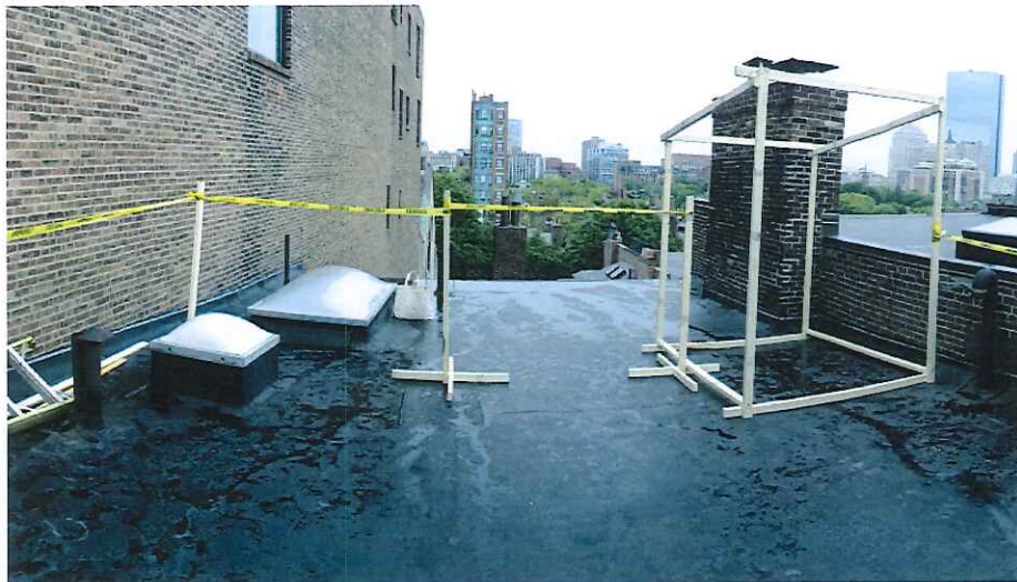
South Facing View
