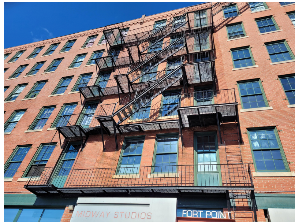
FIRE ESCAPE A TO BE REPLACED IN KIND
