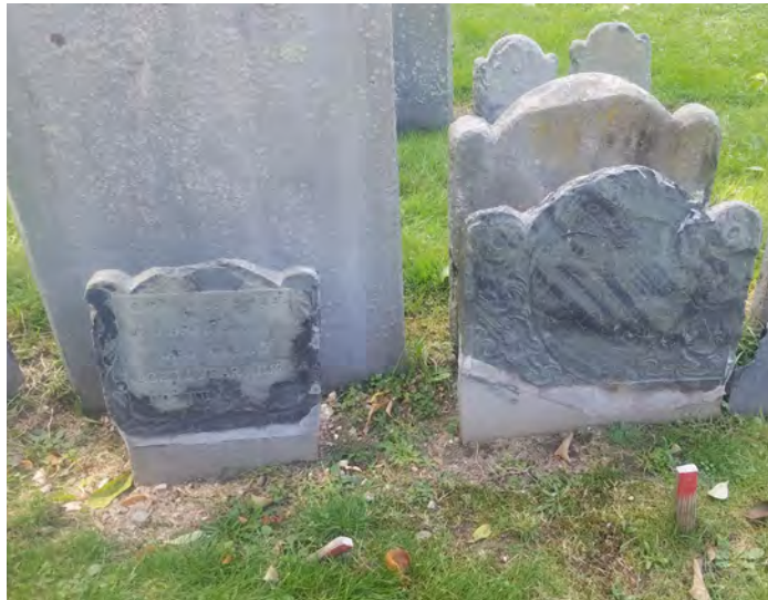
The two gravestones in the foreground were missing the bottom part of the headstone. The conservator added extensions made of concrete to lengthen the headstone so the full epitaph could be above ground.
