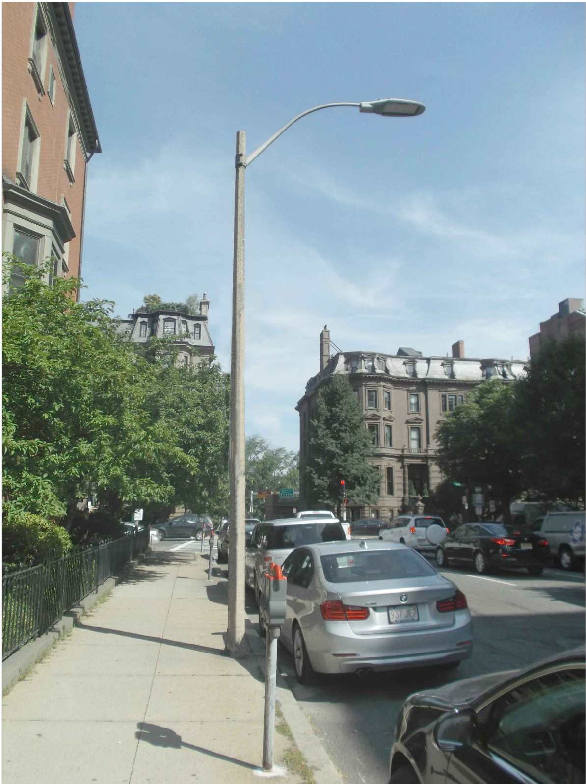
STANDARD CONCRETE LIGHT POLE EXISTING CONDITIONS - EXHIBIT X-18
