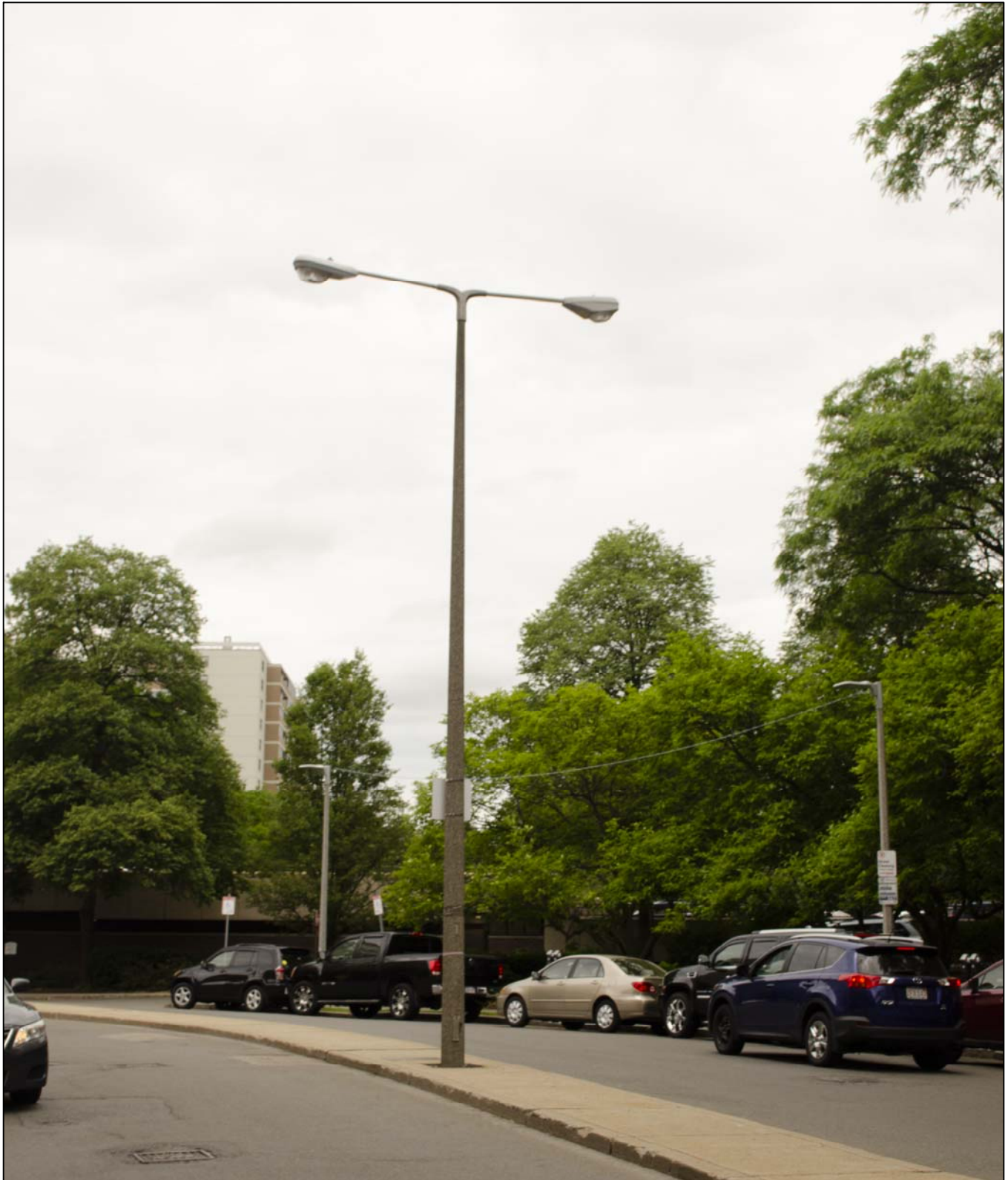
STANDARD CONCRETE LIGHT POLE - DOUBLE STRAIGHT LUMINARY FIXTURE EXISTING CONDITIONS PHOTOGRAPH - EXHIBIT X-1
