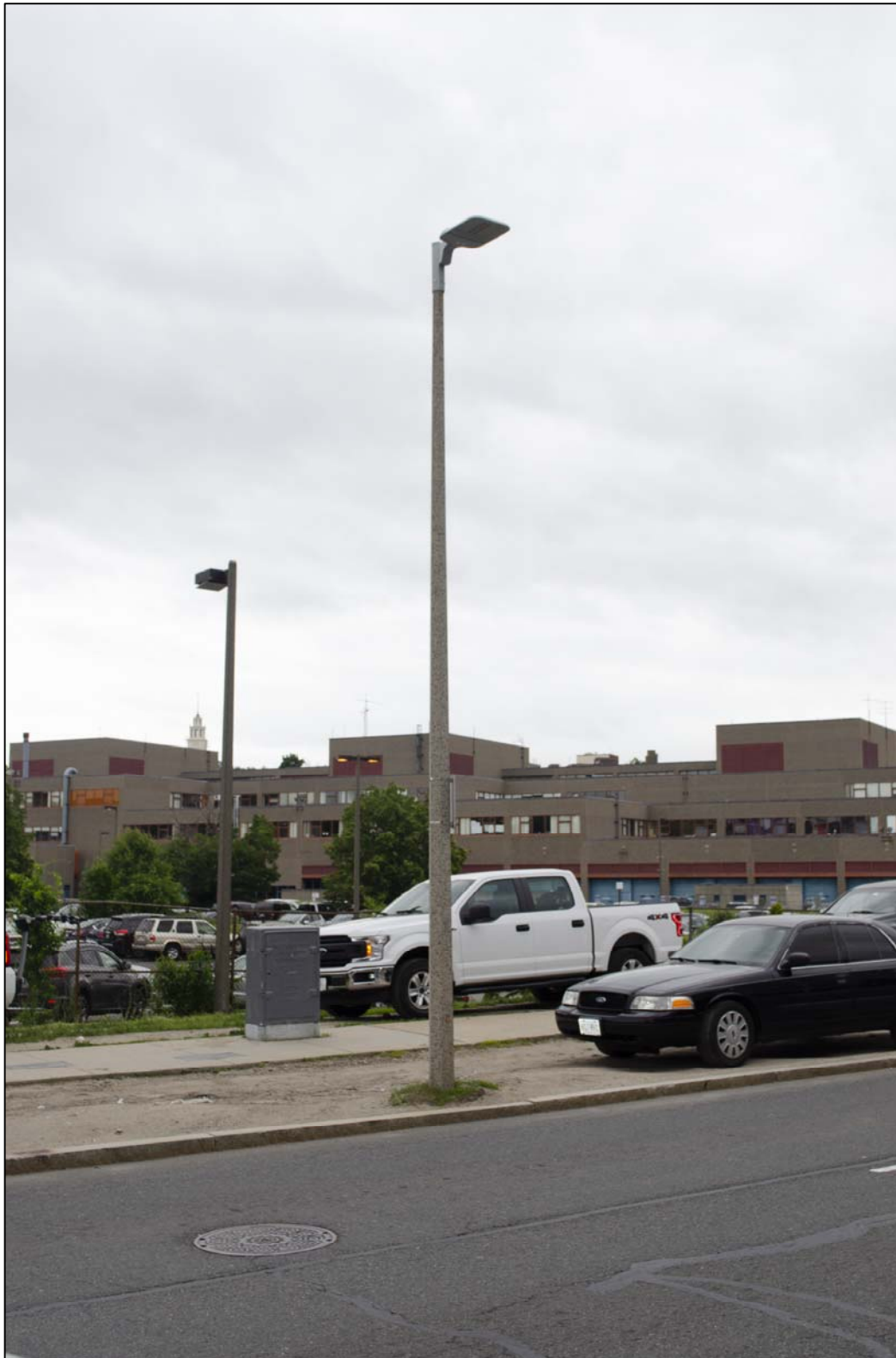
STANDARD CONCRETE LIGHT POLE - AERIATA LUMINARY FIXTURE EXISTING CONDITIONS PHOTOGRAPH - EXHIBIT X-1
