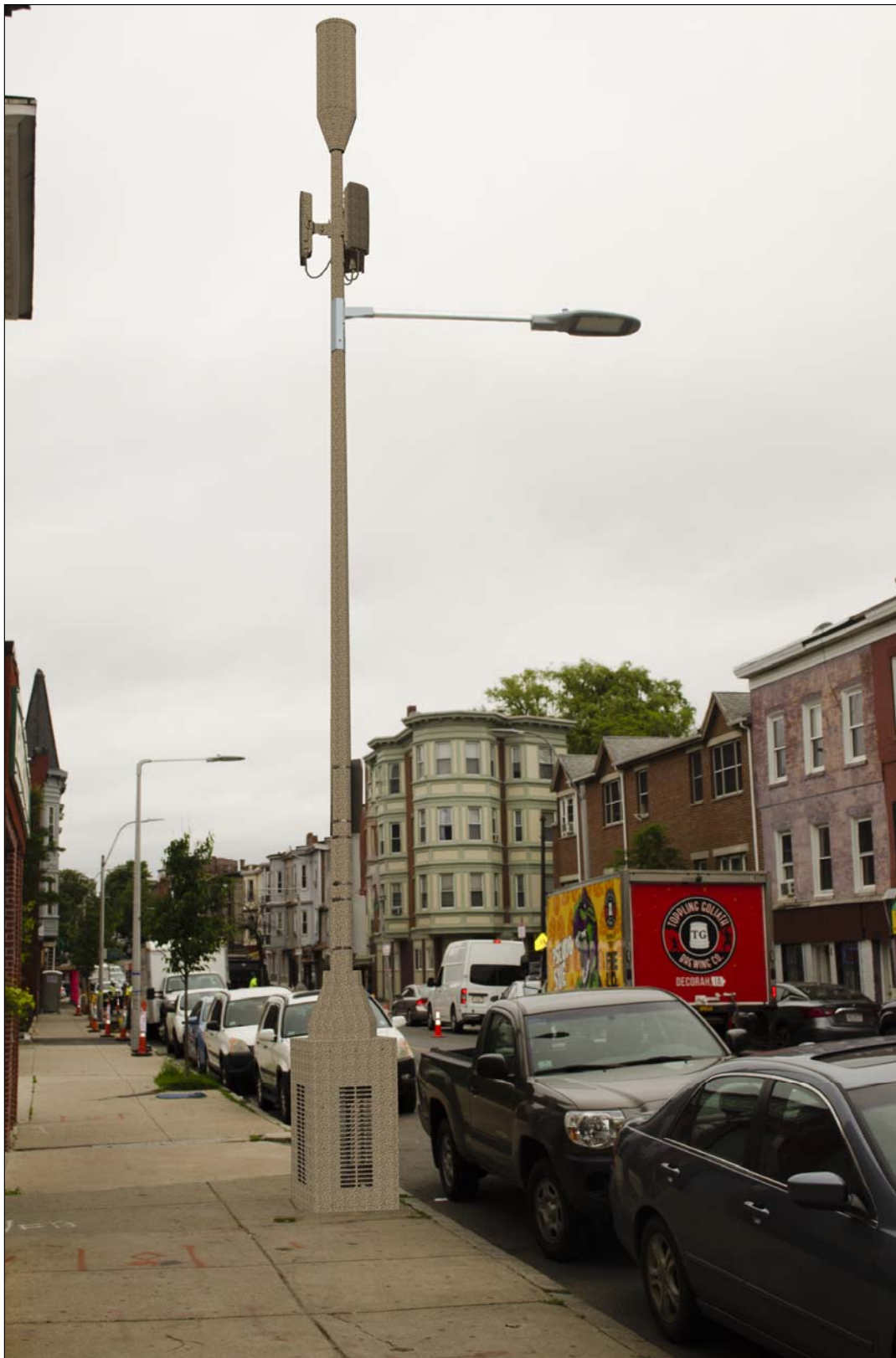
STANDARD CONCRETE LIGHT POLE - EXISTING COBRA LUMINARY FIXTURE PROPOSED STRAIGHT LUMINARY FIXTURE PHOTOSIMULATION - EXHIBIT X-1A
