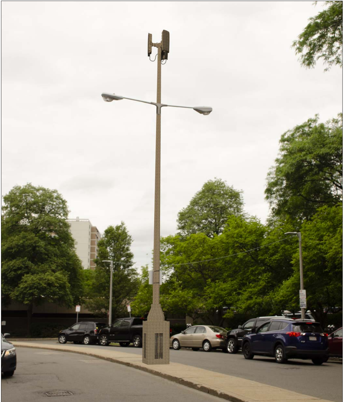
STANDARD CONCRETE LIGHT POLE - DOUBLE STRAIGHT LUMINARY FIXTURE PROPOSED PHOTOSIMULATION - EXHIBIT X-1C
