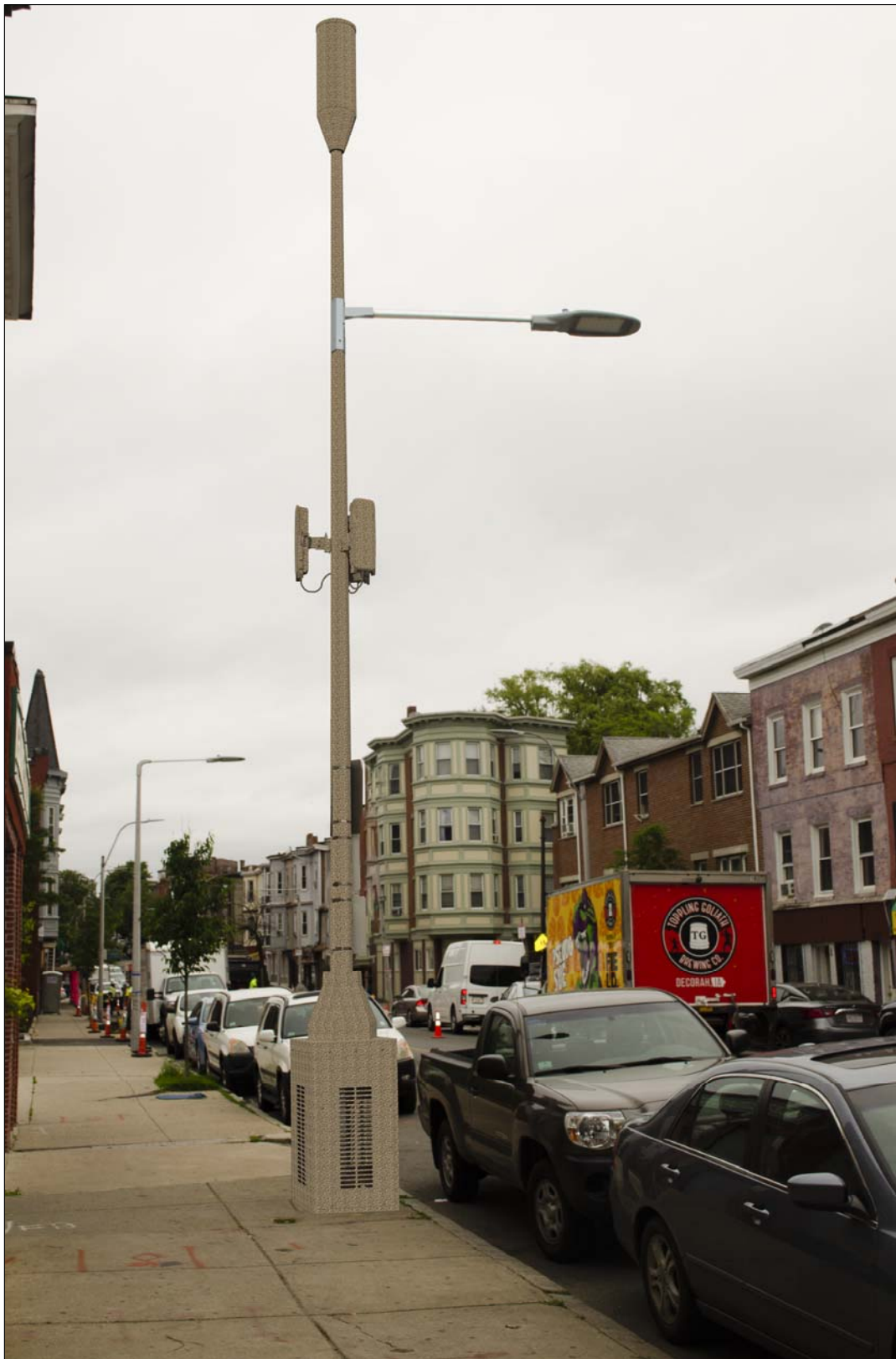
STANDARD CONCRETE LIGHT POLE - EXISTING COBRA LUMINARY FIXTURE PROPOSED STRAIGHT LUMINARY FIXTURE PHOTOSIMULATION - EXHIBIT X-1B
