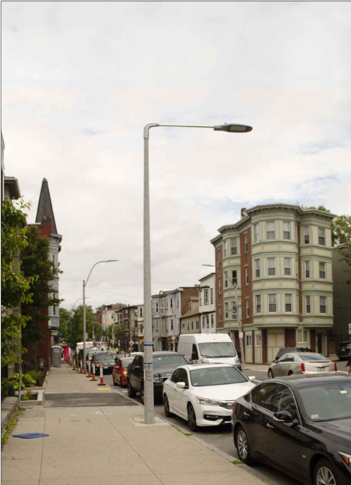
STANDARD CONCRETE LIGHT POLE - STRAIGHT LUMINARY FIXTURE EXISTING CONDITIONS PHOTOGRAPH - EXHIBIT X-3
