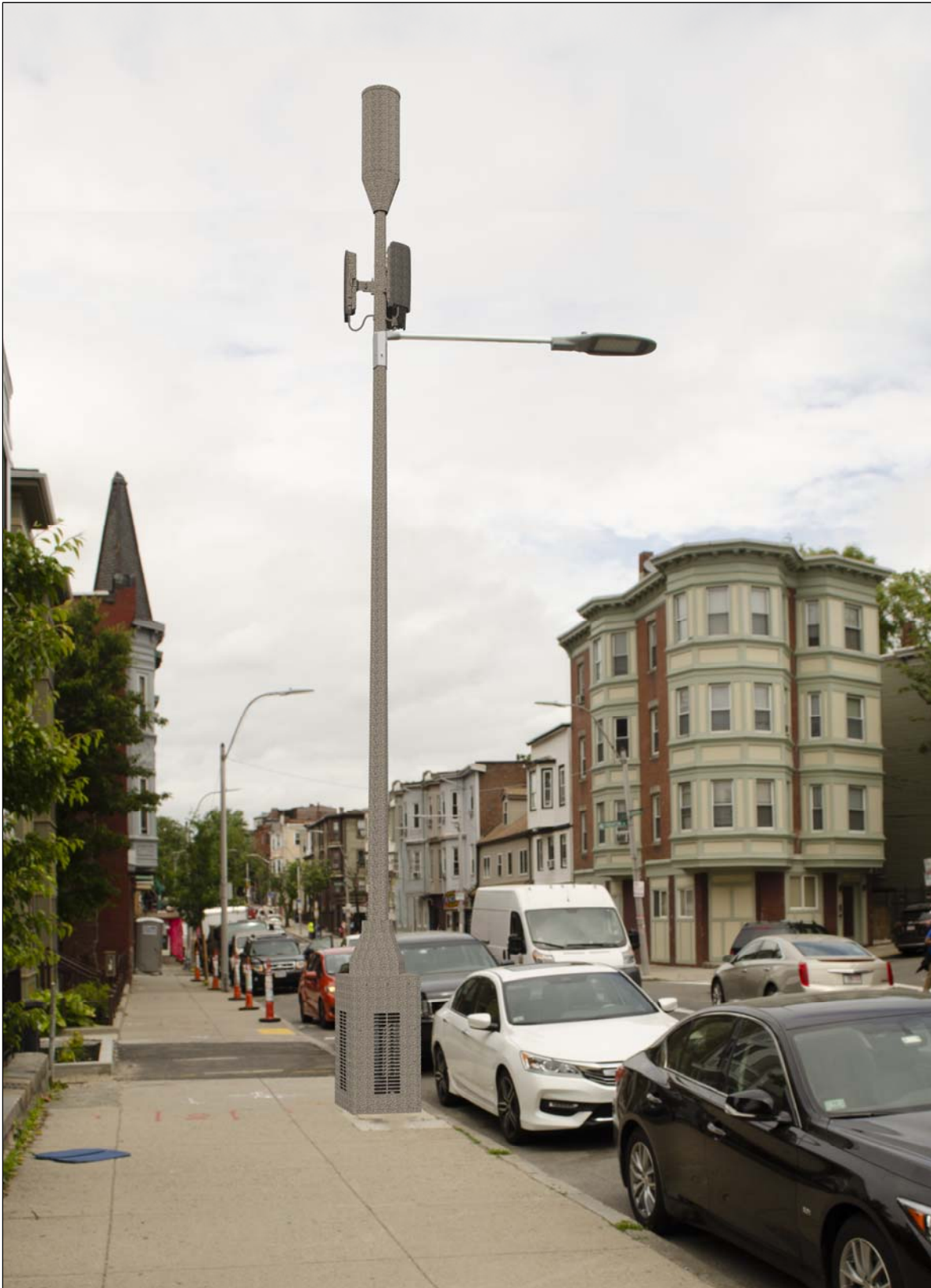
STANDARD CONCRETE LIGHT POLE - STRAIGHT LUMINARY FIXTURE PROPOSED CONDITIONS PHOTOSIMULATION - EXHIBIT X-3A
